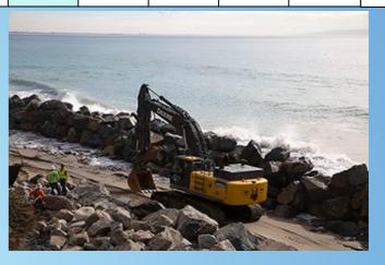
This rock barrier is being constructed along the coast to prevent beach erosion.
