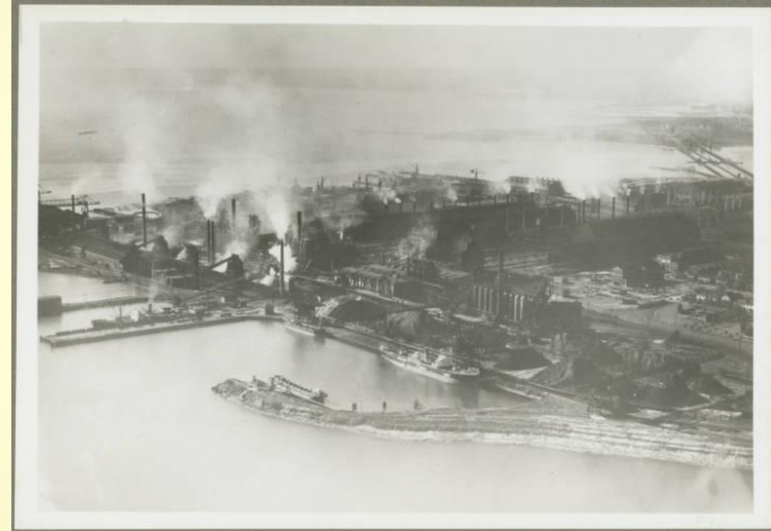
Aerial photograph taken in 1938 of the Bethlehem Steel Company Sparrows Point Yard in Baltimore County. The row of silo-like tanks in the foreground marks the location of the blast furnace, the rows of slender stacks at right angles to the blast furnaces are the open-hearth shops. Also in the foreground is a ship being tied up at the ore dock.
